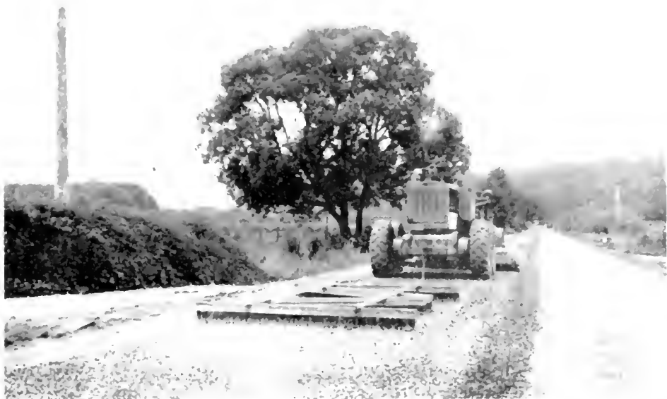
Steel drag broom being towed by motor grader
